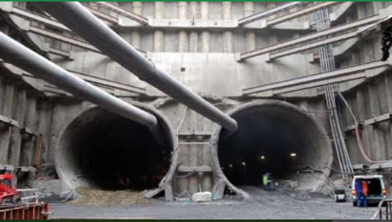
Excavation of side station tunnels
