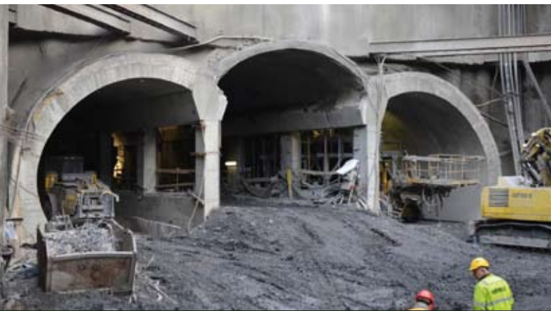
Portal of the mined triple-span metro station
