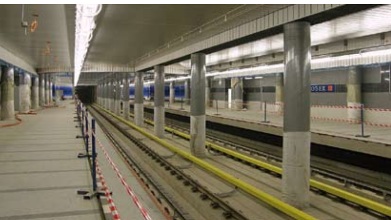
Prosek station - before completion
